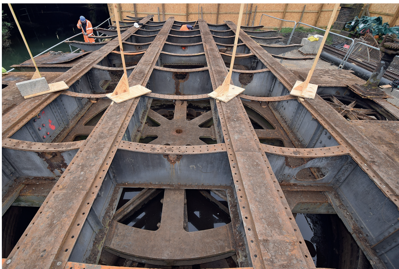
Figure 12: Oxford, Rewley Road Swing Bridge.
