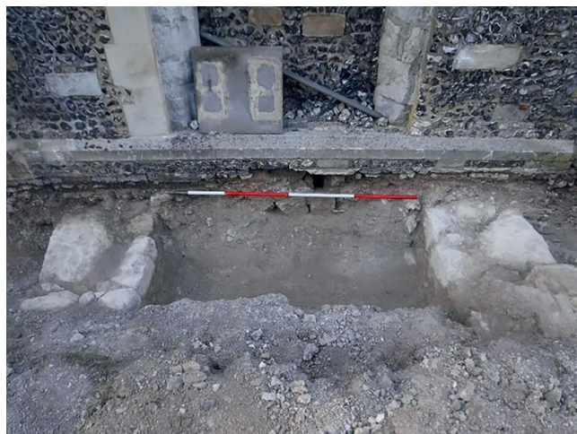
Figure 7: Drayton Beauchamp, foundation of south porch with base of blocked door (Scale = 2m).
