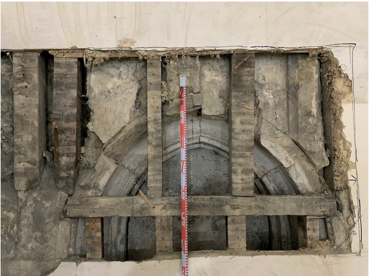
Figure 20: Oxford, Medieval door exposed by renovations at the Old Library, Christ Church (Courtesy of Graham Keevill).
