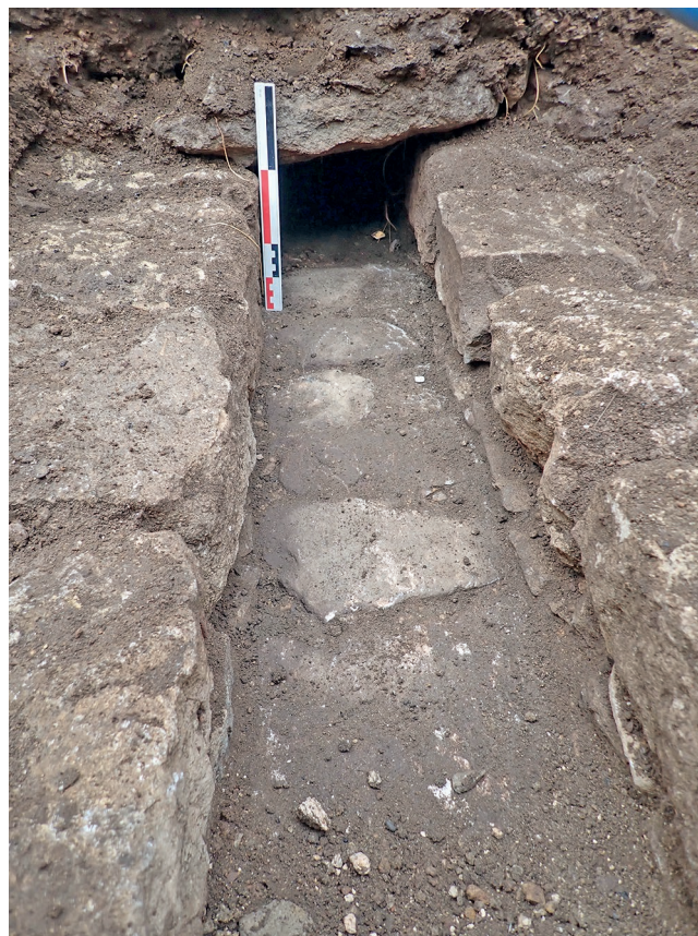
Figure 10: Hertford College, stone lined drain (with capstones removed).
